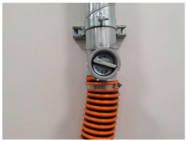
Open the valve for the exhaust just a crack. You will hear a low hiss. The picture above shows this. If the exhaust is opened completely, the fan will pull so much air out of the oven that the heating element will not be able to heat the boards.
